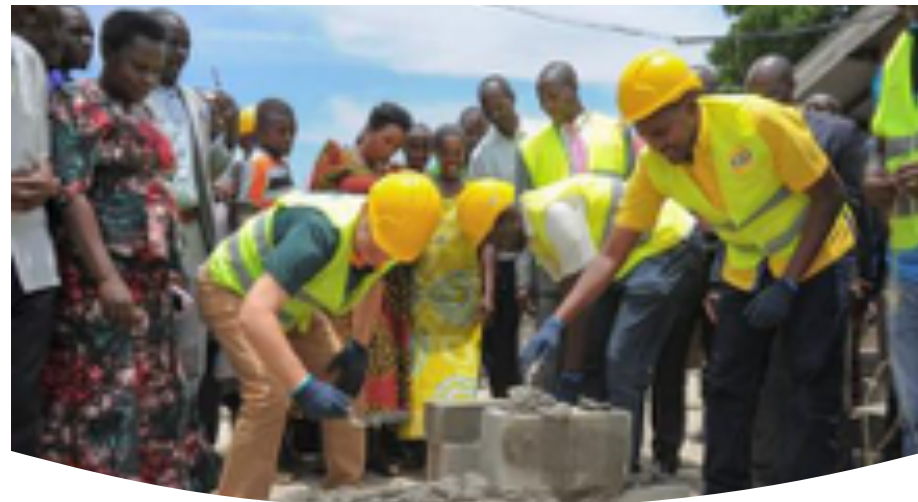
The corporate build day at Bwizi Health Centre
